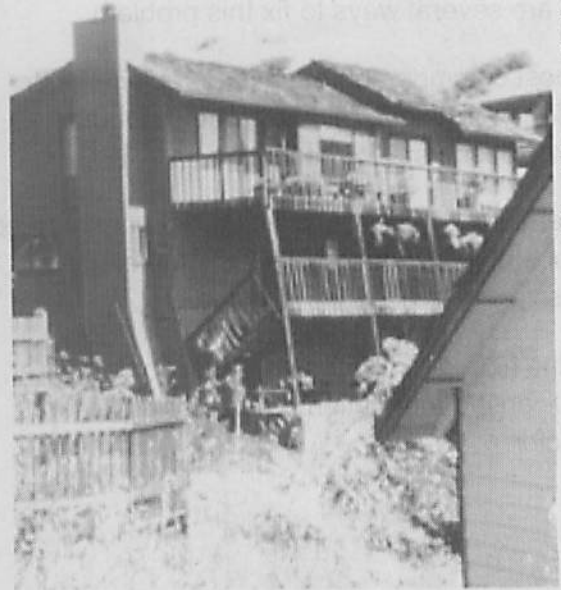
Figure 22 - This hillside home was built on an unbraced tall wall that failed.
