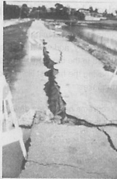
Figure 39 - Lateral Spreading. Loma Prieta Earthquake, October 17, 1989. Lateral spreading damage levee road along the San Lorenzo River.
