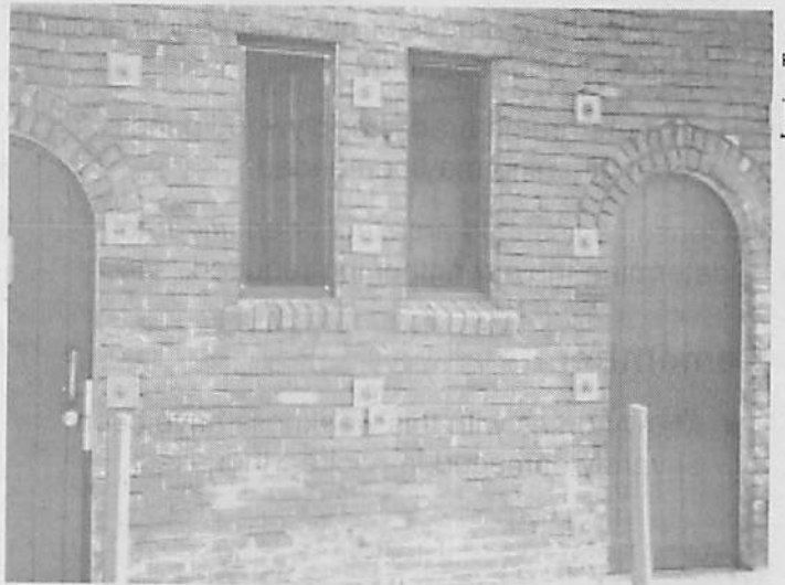
Figure 28 - Bolting of unreinforced masonry wall to steel frame on the inside.
