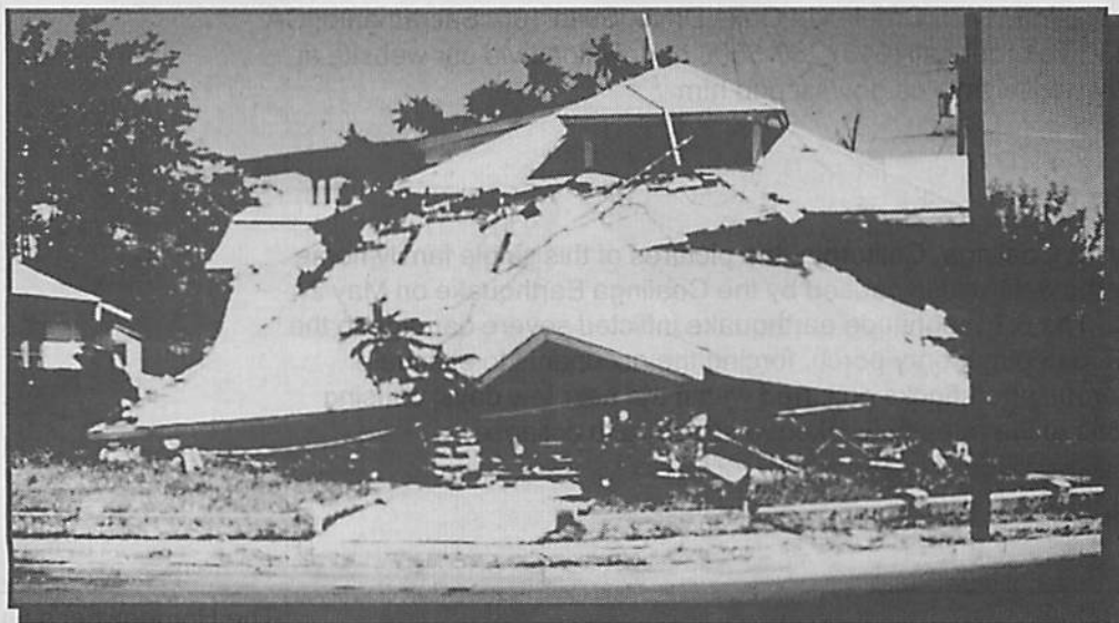
Additional damage from aftershocks
